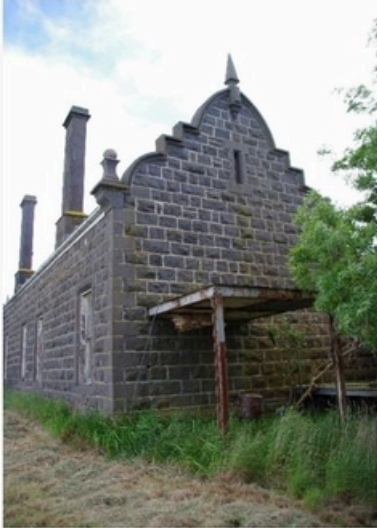
Parapet gables removed from the south side of the house
