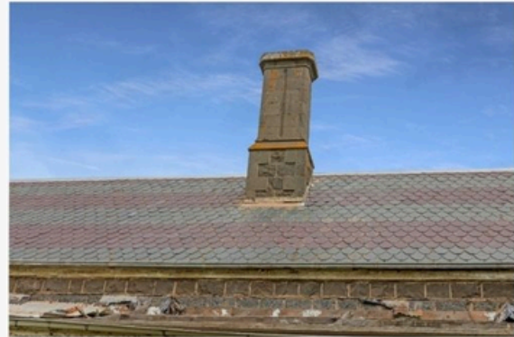
The slate clad roof has two tones of slate laid in a fish scale pattern with wide bands of each colour forming stripes
