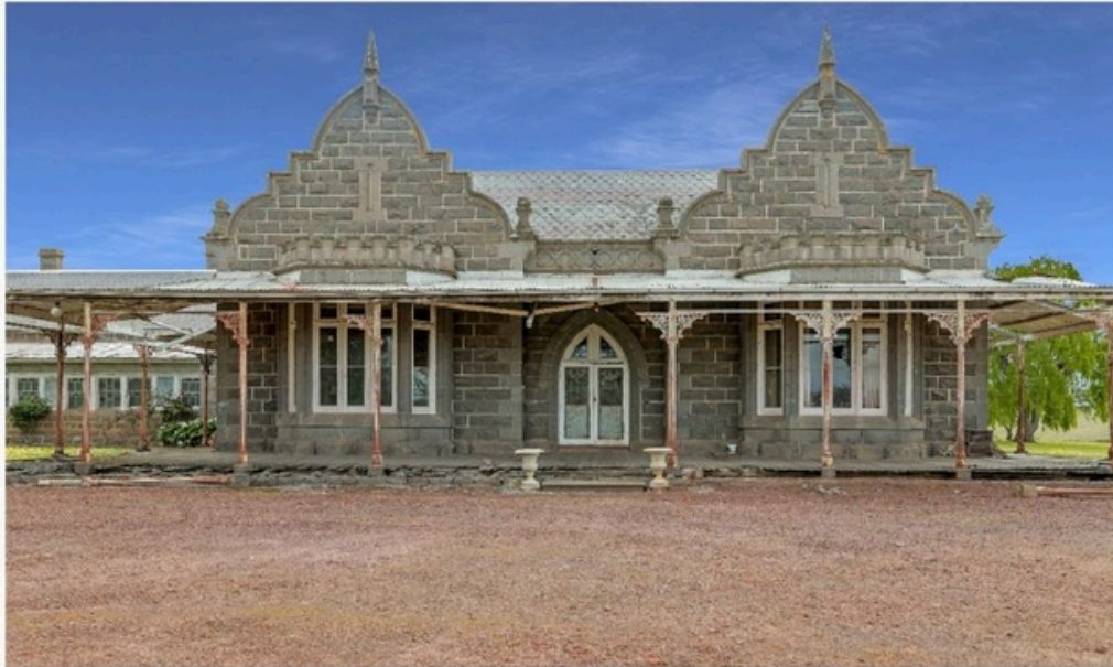
Front of Berrambool showing the bluestone parapets, central keystone, finials and baubles.
